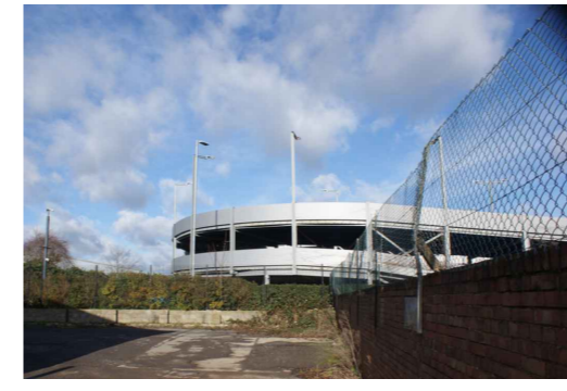
Existing brick wall C Scale NTS
