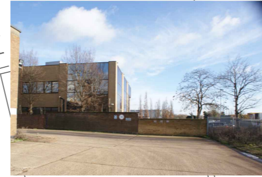
Existing brick wall C Scale NTS
