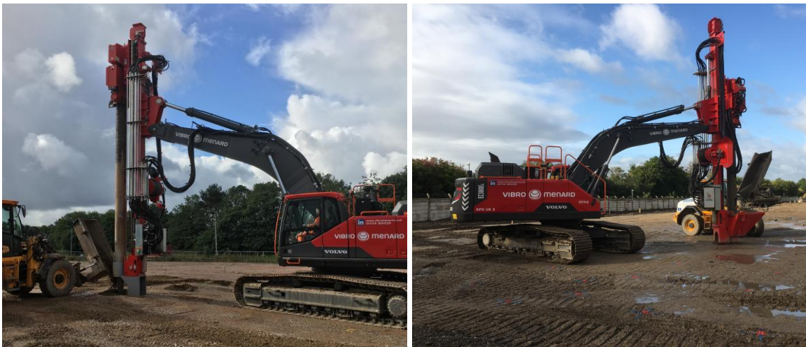
Figure 3 - VSC rig on site (Top Feed – left, Bottom Feed – right)
