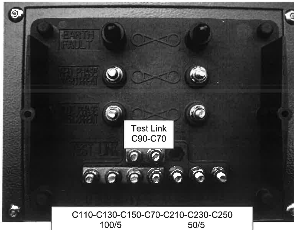
Figure 1. Protection CT ratio selection & terminal identification.
